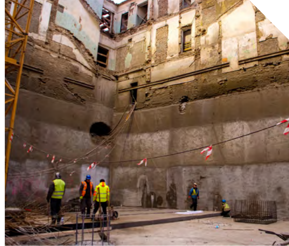
UNDERPINNING OF THE EXISTING STRUCTURES
