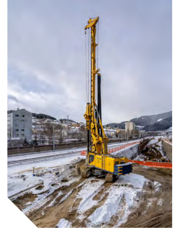
PORTAL: CONSTRUCTION OF BORED PILES
