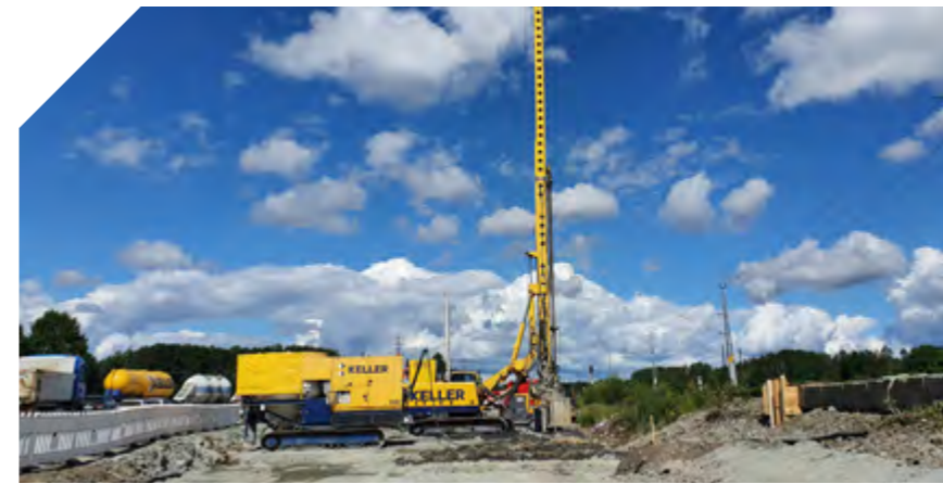
DDSM (DRY DEEP SOIL MIXING) WORKS
