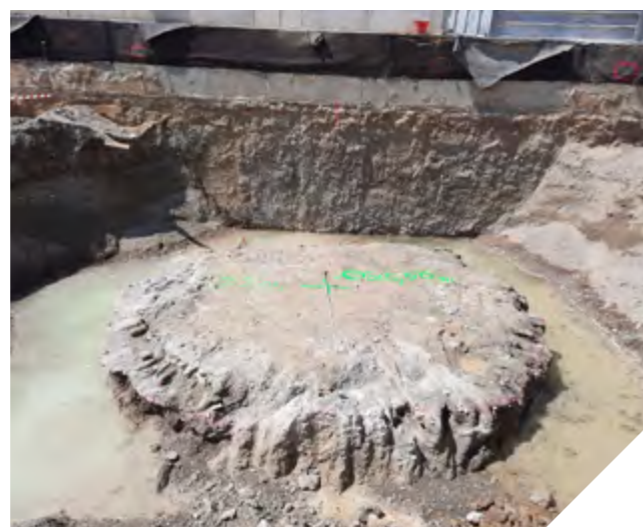
FIELD TEST (SINGULAR COLUMN DIAMETER 550 CM)
