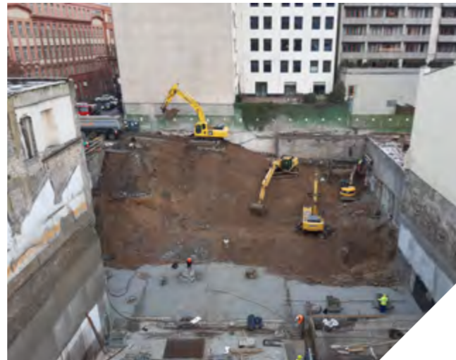
EXCAVATION OF THE PIT
