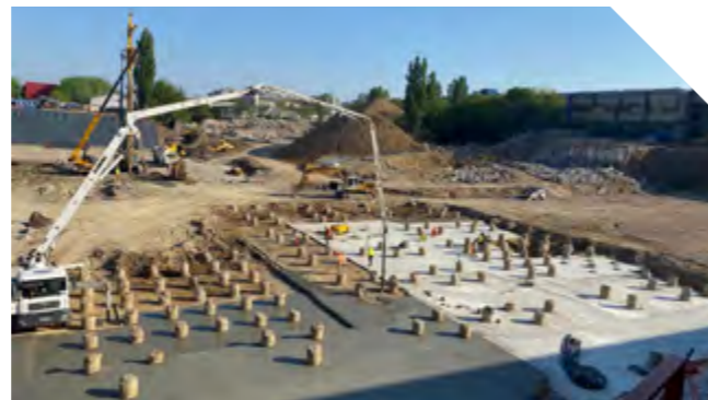
EXECUTION OF CFA PILES
