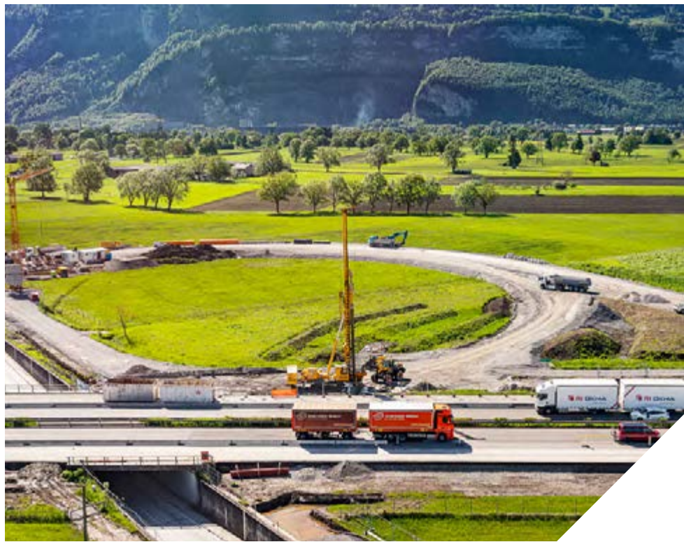
WORKS VERY CLOSE TO THE HIGHWAY
