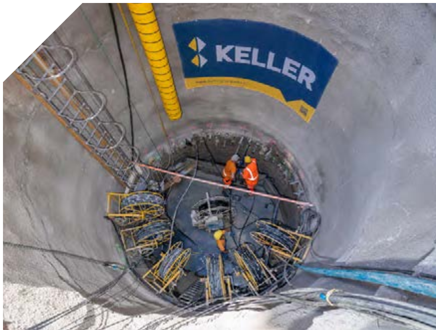
PLACEMENT OF THE DOUBLE PACKERS
