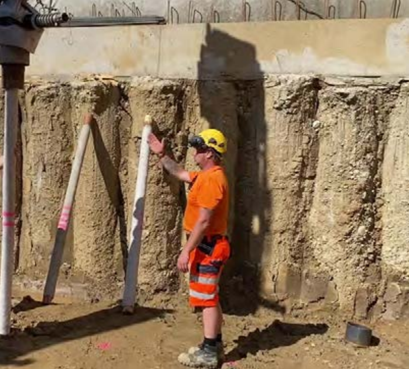
INITIAL TESTS FOR DRIVING POLYMER CEMENT-COATED, impregnated timber piles.
