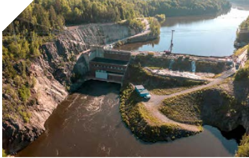
REPAIR WORKS AT THE MELO HYDROPOWER PLANT in Nokia, Finland
